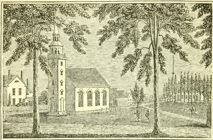
Southwest view of the Episcopal Church, Stratford.
